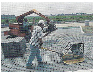
Aggregate base is spread and compacted; pavers are delivered ready to install. After placement of bedding course, joints and/or openings are filled with small aggregate and the pavers are compacted. Joints may be filled mechanically as shown.
