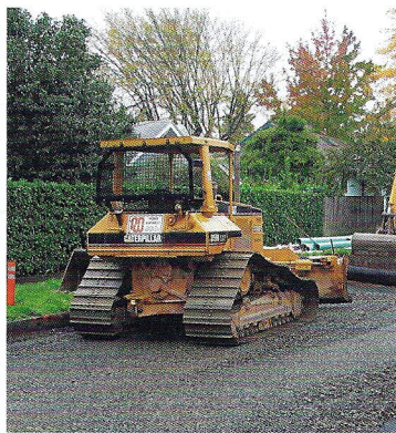
Prepared subgrade for 20,000 sf (2000 m 2 ) Portland, OR street retrofit with PICP
