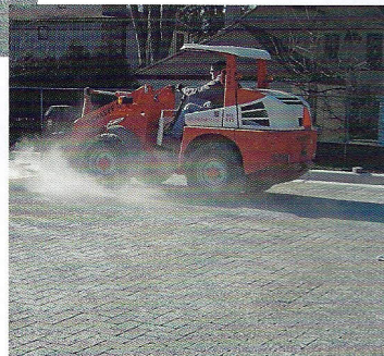
Aggregate base is spread and compacted; pavers are delivered ready to install. After placement of bedding course, joints and/or openings are filled with small aggregate and the pavers are compacted. Joints may be filled mechanically as shown.
