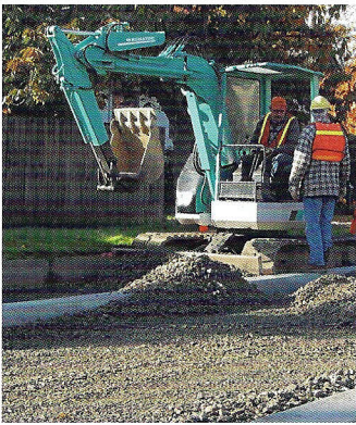
Prepared subgrade for 20,000 sf (2000 m 2 ) Portland, OR street retrofit with PICP
