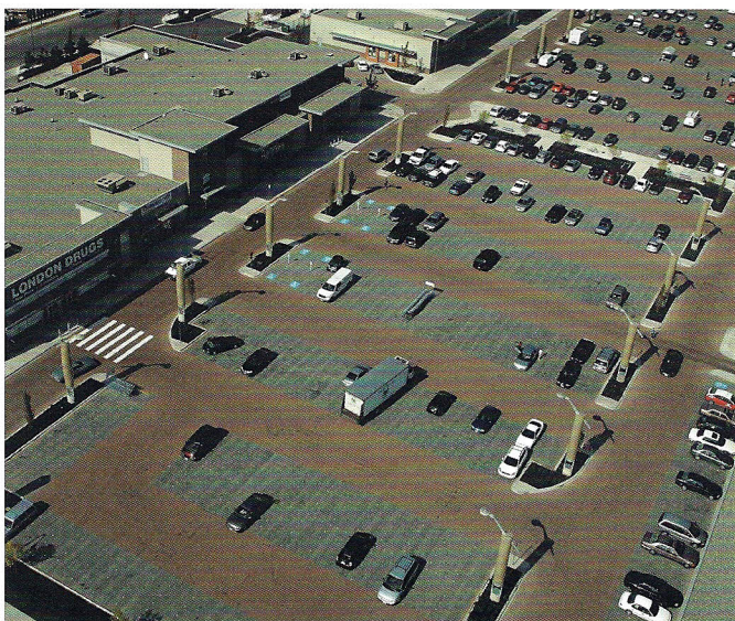
350,000 sf (3.2 ha) of PICP at a Burnaby, BC shopping center infiltrates runoff from roofs.
