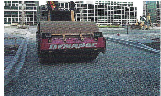
Aggregate base and subbase are spread and compacted; pavers are delivered ready to install. After placement, joints and/or openings are filled with small aggregate. Then pavers are compacted.
