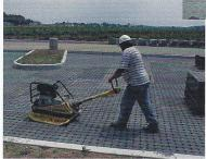
Mechanical installation equipment accelerates construction; typical 5,000 sf (500 m<sup>2</sup>)/ machine/day.
