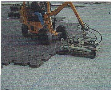
**Mechanical installation equipment accelerates construction; typical 5,000 sf (500 m<sup>2</sup>)/ machine/day.**
