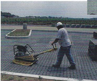
**After placement, joints and/or openings filled with small aggregate and pavers are compacted.**
