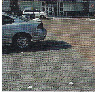
Stormwater treated in drive and parking space areas in Vancouver, BC shopping center.
