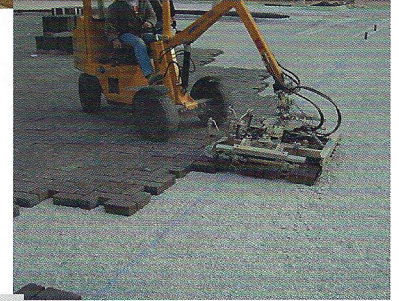
Mechanical installation speeds construction.
