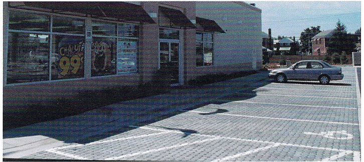
Permeable interlocking concrete pavement at this fast food restaurant in Baltimore, MD treats stormwater before entering the Chesapeake Bay.
