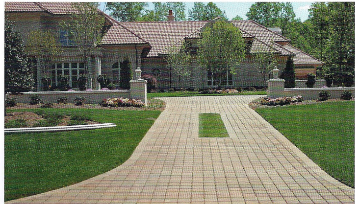
PICP driveway in NC creates an attractive and environmentally responsive entrance.
